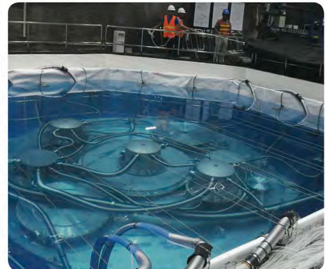
That was fast! Construction of China's Daya Bay Reactor Neutrino Experiment began in 2007. With 2 months' worth of data, it scooped competitors in Japan, France, Korea, and the United States.
